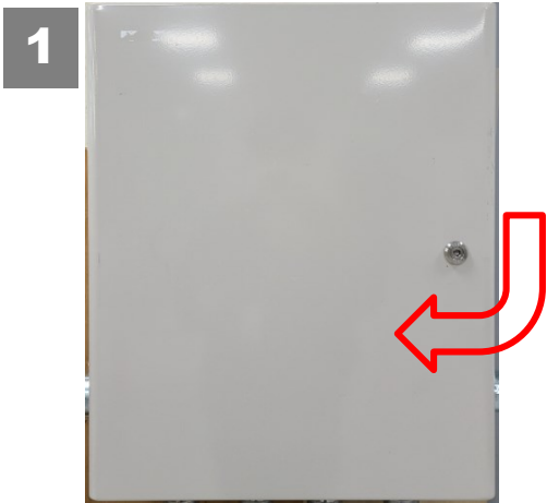
Open front cover with Hex wrench 8mm
